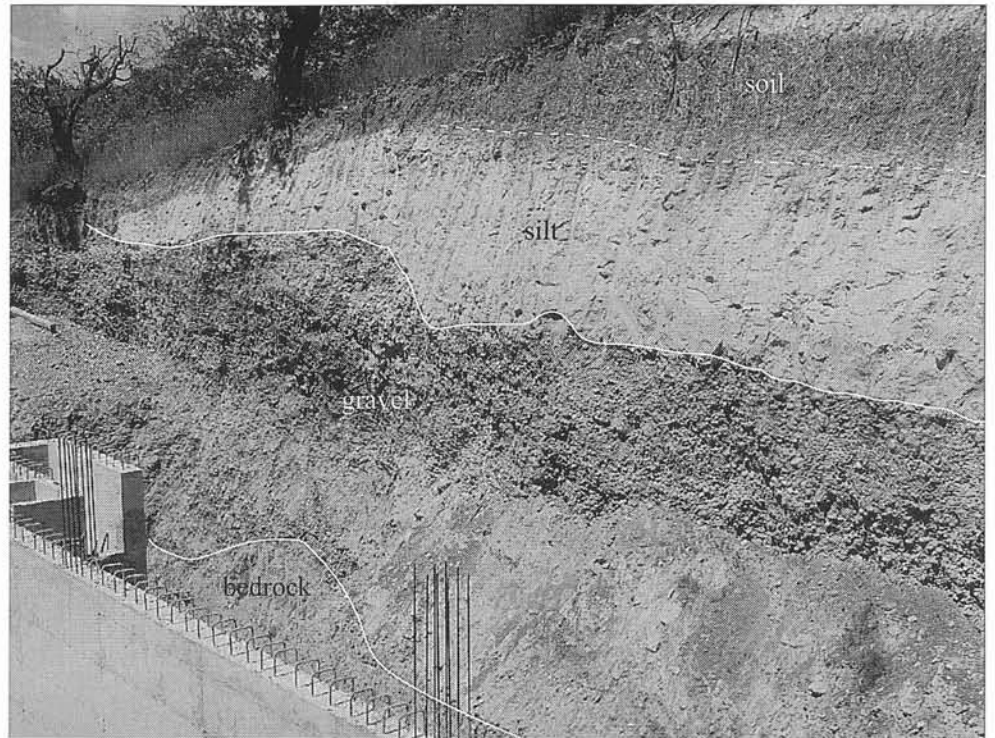
FIG. 8 - Typical terrace section.
