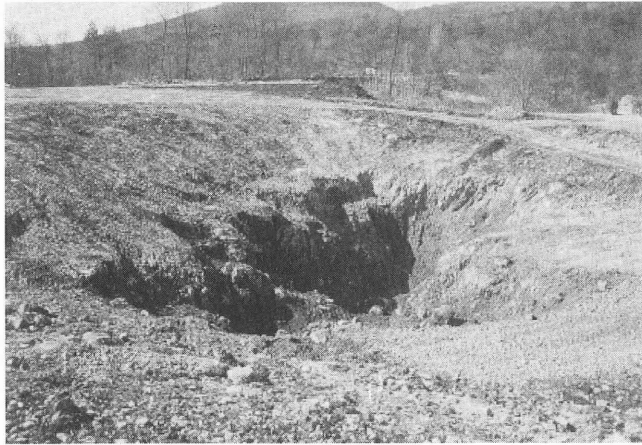
FIG. 2 - A doline which was formed above an infilled shaft. During the highway construction, the top soil was removed and the double structure of the doline was exposed. The upper part was formed by slope processes and solution in the subcutaneous zone of the karst. The lower, in cross section more irregular part is the remnant of a solution shaft filled with sediments. The circumference of the doline is clearly distinguished from the irregular cross section of the shaft which is filled with loam.
