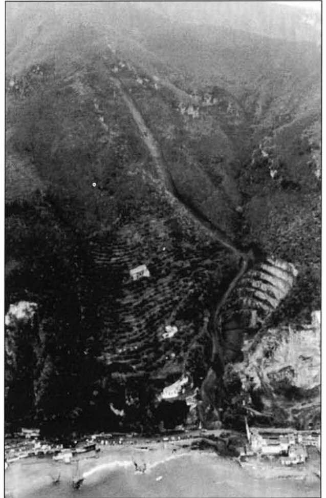
FIG. 8 - The landslide occurred at Pozzano on January 10, 1997 in a photo taken a few days after the event (courtesy of A. SANTO).
