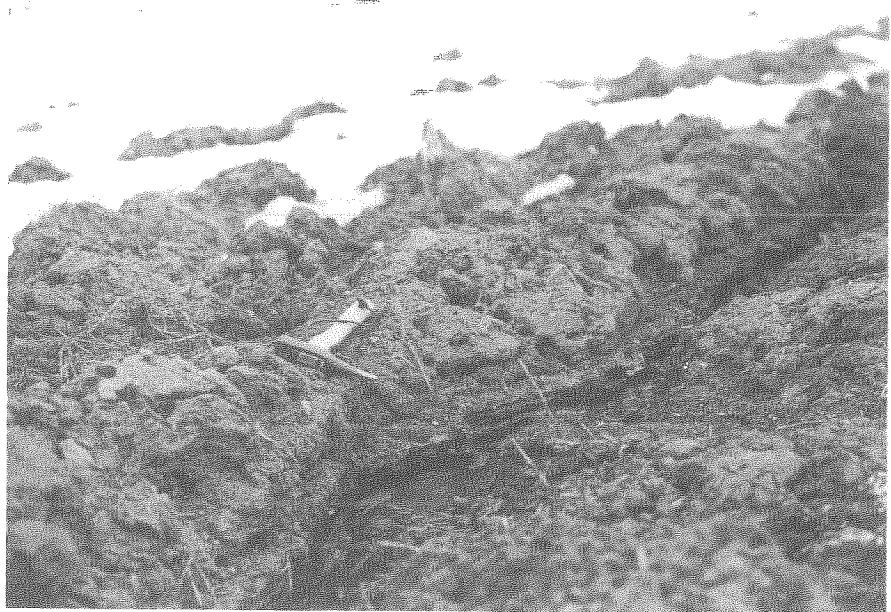
FIG. 6 - Ground water seepage from damaged drainage pipes have lateral thermoerosional effects on the rill walls.
