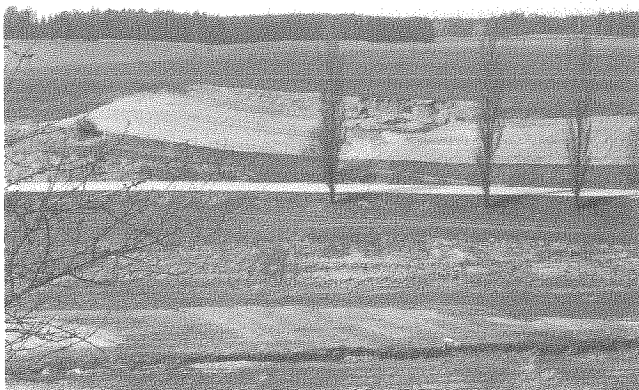
FIG. 20 - Flood bank markings after the flood in the central part of the short catchment. The slope of the terrace on the dell floor was soaked with water and suffered planar slide (Kozlov, April 1988).
