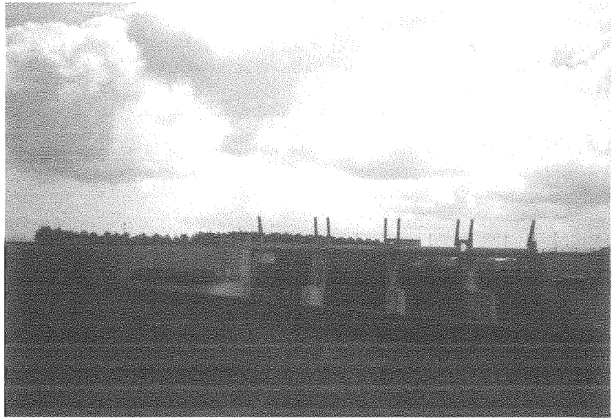
FIG. 4 a - The flow-regulation system of the Scolmatore, near Pontedera.
